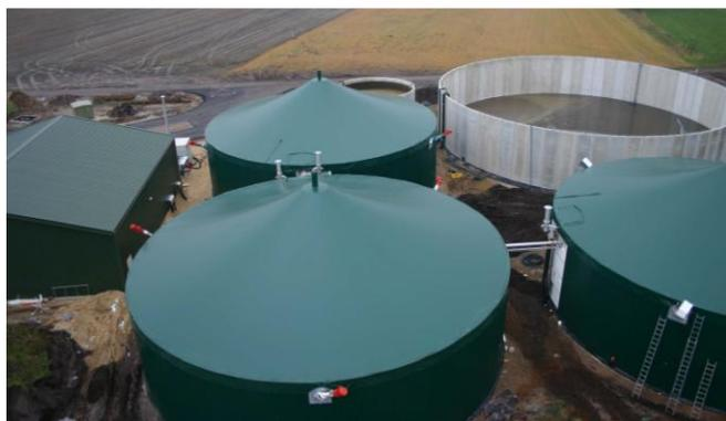
The Biogas is converted to electricity by a co-generation unit. The heat energy which accrues at the same time is used for self consumption and the surplus is utilized in a container for the drying of fire wood.
