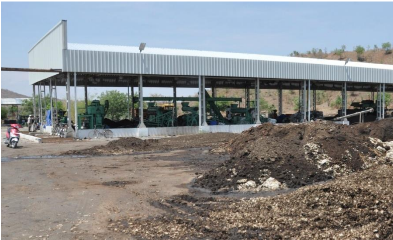
The compost part of the Jalgaon plant
