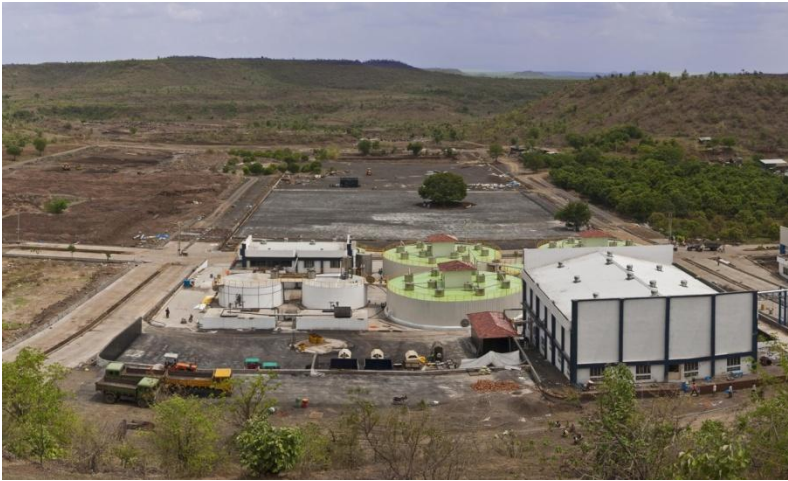
The Biogas plant under construction
