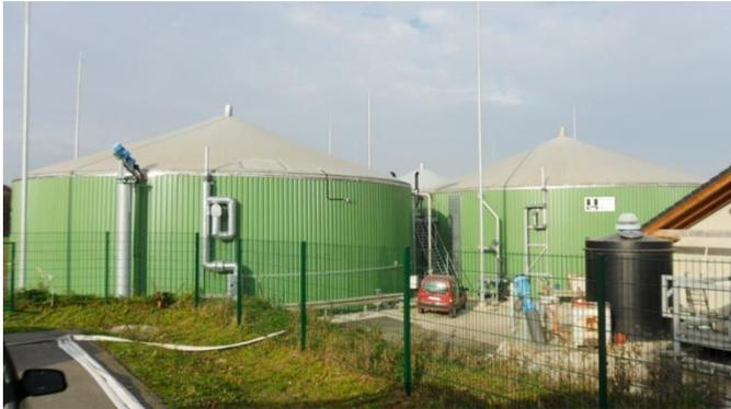
The biogas plant Gera, township Aga, was completed in 2011 as a typical agricultural biogas plant with Main Fermenter, post fermenter and storage tank for digestate.
