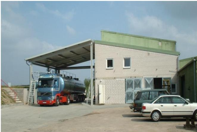
The Biodiesel Bokel GmbH was followed from a typical agricultural distillery cooperative. The former grain distillery was rebuilt to a biodiesel production with a capacity of 10,000 t of biodiesel per year. The big advantage for the investors was that many apparatus and devices could be reused or refit for the biodiesel production.
